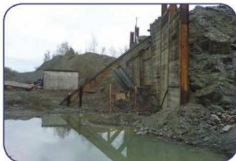
▲ Remnants of the stone crusher loading point stone was tipped from the trucks into the stone crusher at this point ▼
