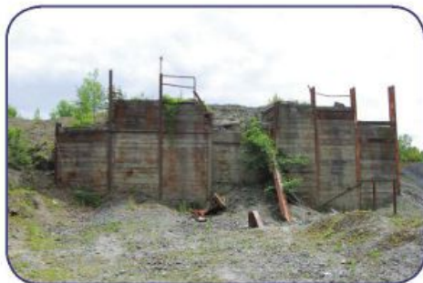
▲ Remnants of the stone crusher loading point stone was tipped from the trucks into the stone crusher at this point ▼
