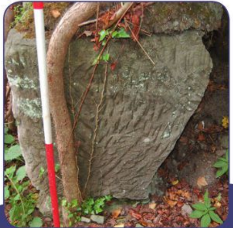
▲ All of the quarry faces show pick marks made by the workers, this is one example
