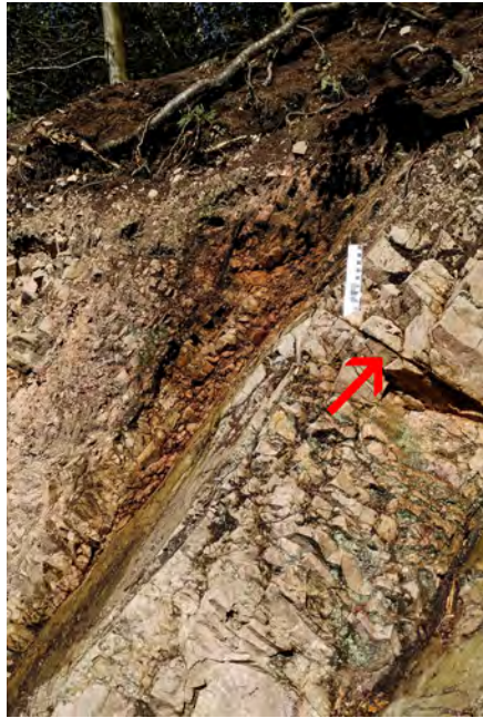
Figure 18 – Below the fissure ①, a well-defined, persistent joint is filled with sandy material, comparable to the matrix of the fissure infill. This suggests that it had been opened before the fissure filled.
