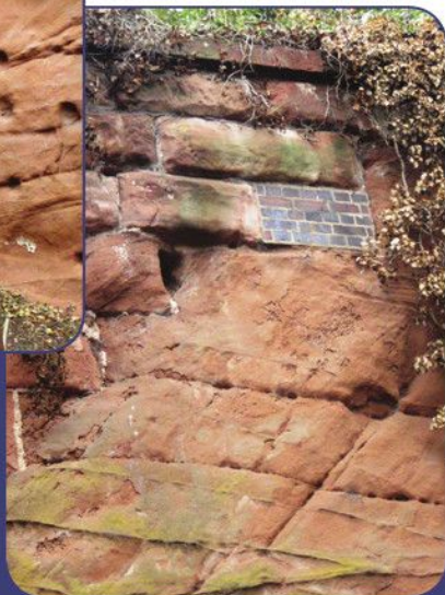
▶ New Red Sandstone used in viaduct with brick repair
